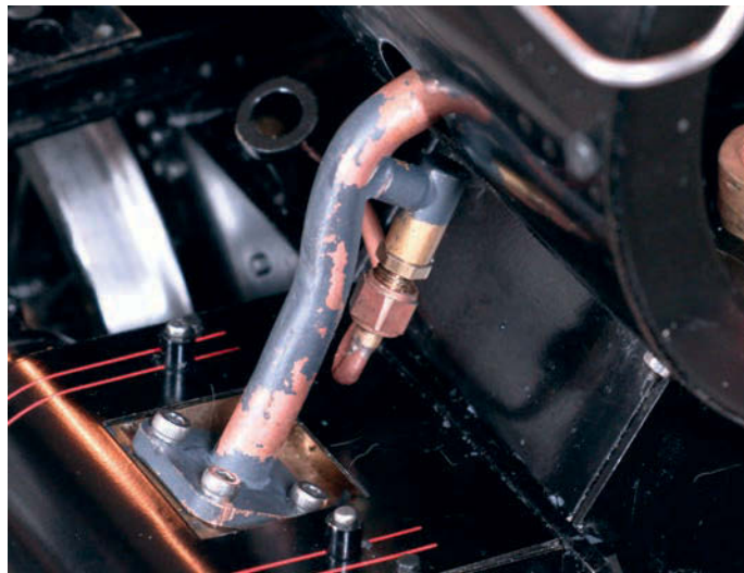
Photo 14: Steam pipe from cylinder.
