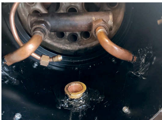
Photo 15: Sealing the pipework with more Fireweld.
