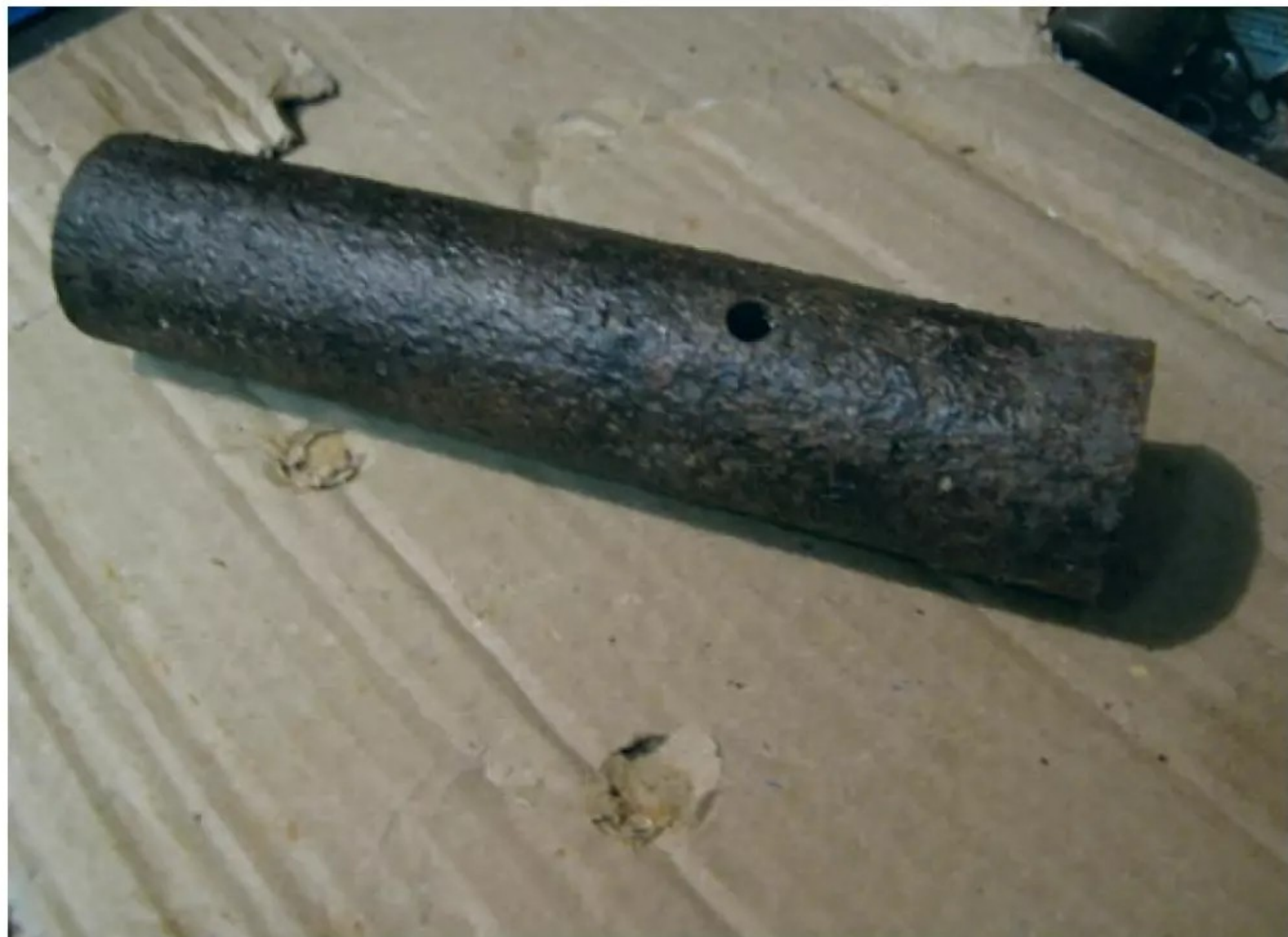
Photo 24: The rusty water pipe.
