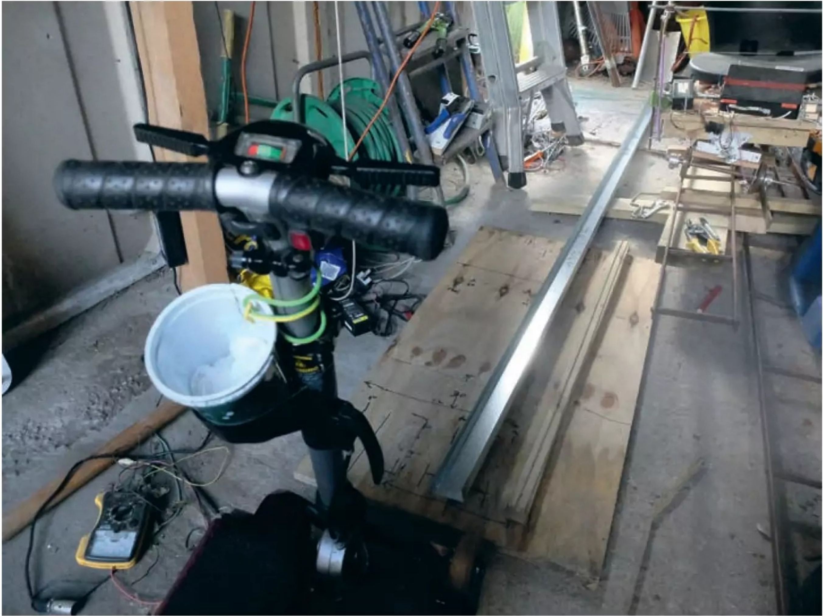
Photo 5: Scooter ramp preparation.
