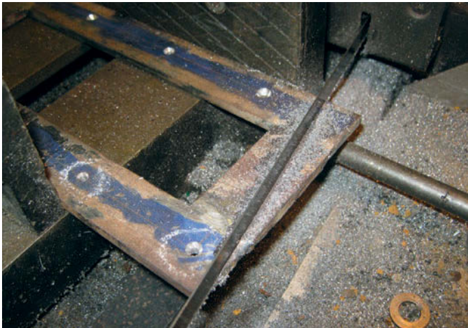
Photo 7: Trimming the end of the frame.
