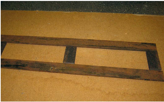
Photo 4: Laid out as they will be welded.
