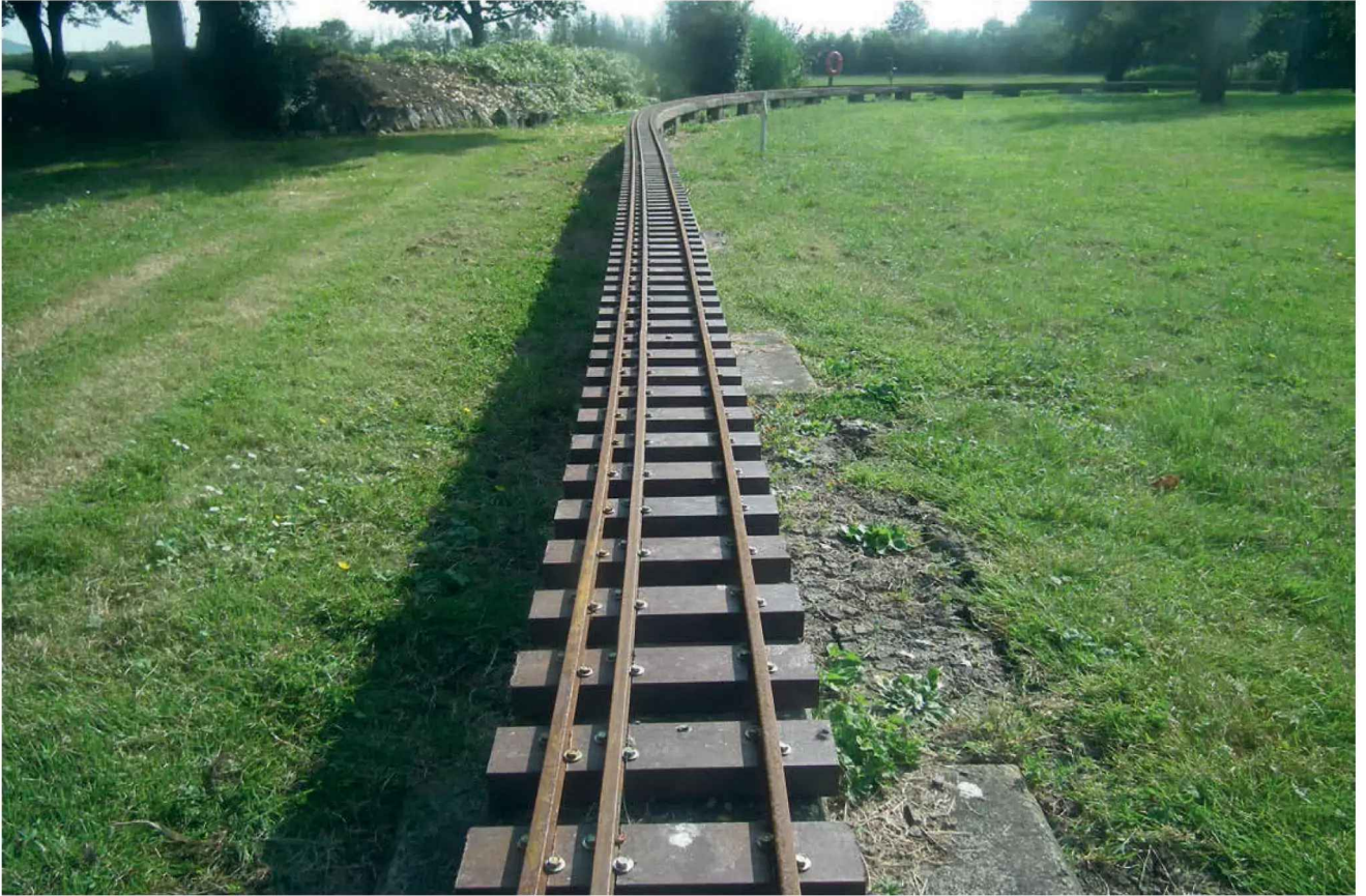
The track with its new sleepers heads into the distance at West Huntspill MES.
