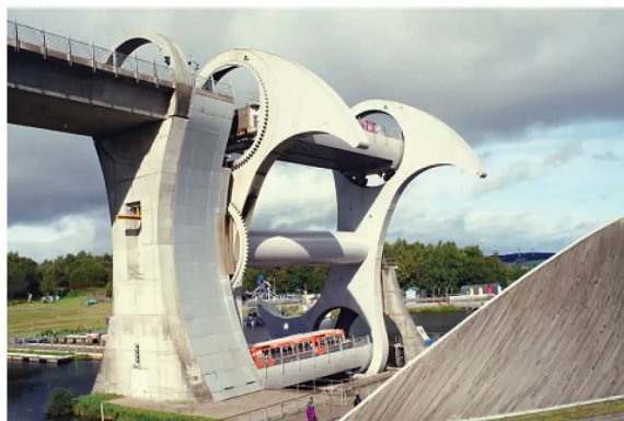
Photo 9: Gondola with boat seen from bank near the start of the lift. It is almost completely silent in operation.
