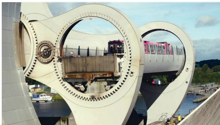
Photo 10: The gondola nears the halfway point of the lift showing the gear wheels.
