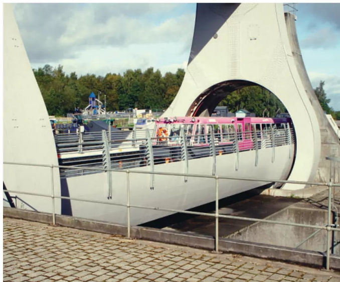
Photo 8: Boat enters lower gondola ready for lift
