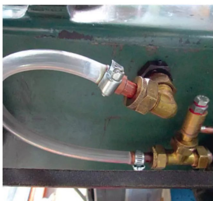
Photo 20: M16 locating bolt in situ, short length of flexible pipe.
