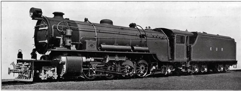
2-8-2 type Locomotive, Kenya & Uganda Railway, built by Robert Stephenson & Co. Ltd., Darlington.
