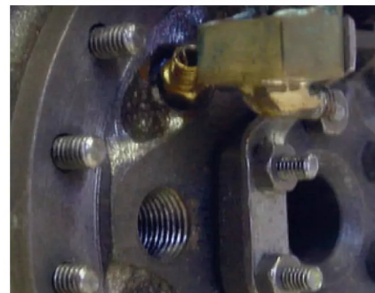
Photo 178: An end cover fitted.
