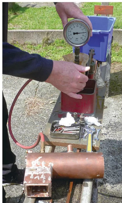
Photo 118: Boiler test day.
