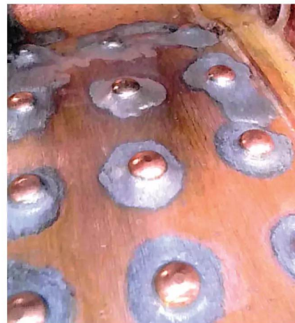
Photo 117: An inspection of the inner firebox by borescope.
