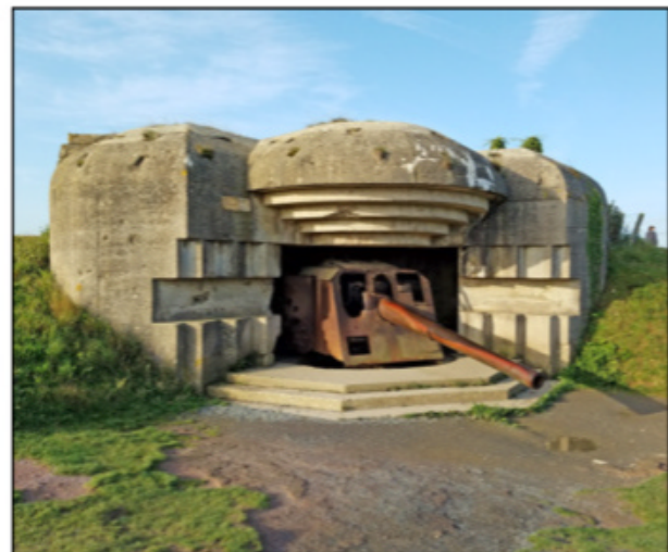
Crumbling visual reminders, like this German gun and bunker, remain atop the bluffs.
