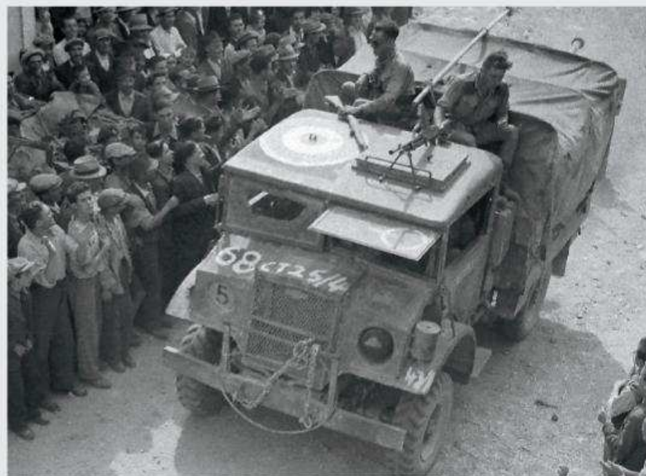
Chevrolet C15A 15-cwt GS being used as a 6-pounder tractor by the Carleton and York Regiment antitank platoon. The pole across the top is the rammer staff for the gun. I don't know why the serial number on the service marking is so large and crude.
