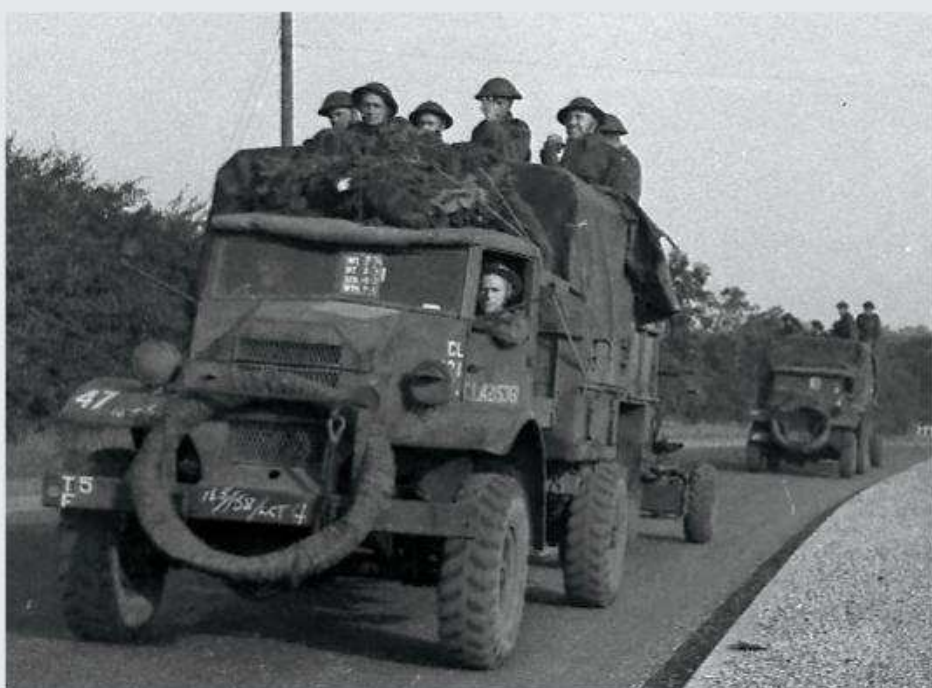
Cab 12 Chevrolet C30 30-cwt light anti-aircraft tractor towing a 40mm Bofors gun. Likely from the 2nd LAA Regiment; the unit has been in a beach landing exercise, as shown by the chalked LCT marking on the bumper and vehicle-dimension chart on the windshield. England, 1942.
