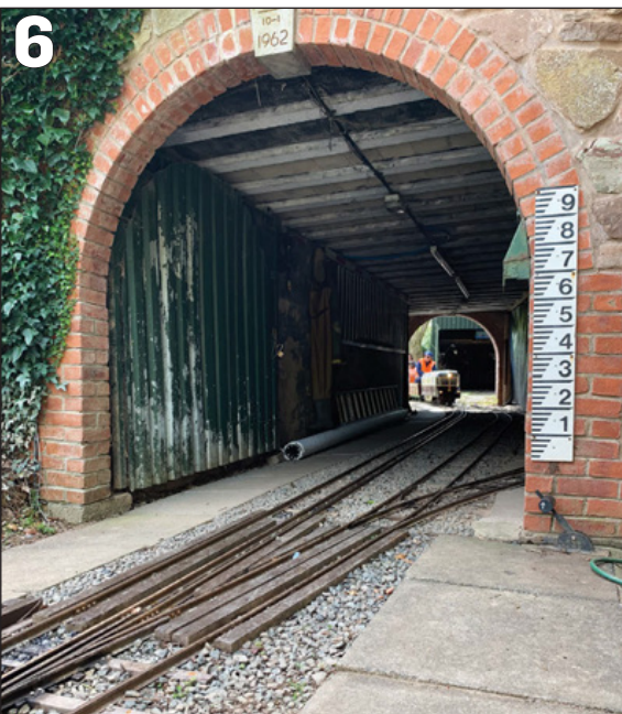
PHOTO 06: Tunnel exit – note the scale on the right-hand wall that allows the depth of flooding within to be judged!
