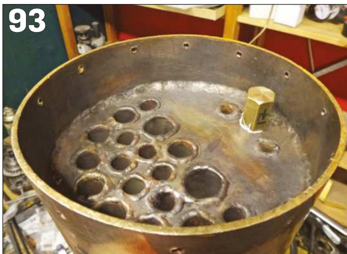
PHOTO 93: Finished job – the boiler tubes are now welded to the front tubeplate.
