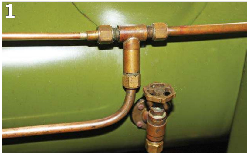
PHOTO 1: External fitting for the vacuum ejector feed .
