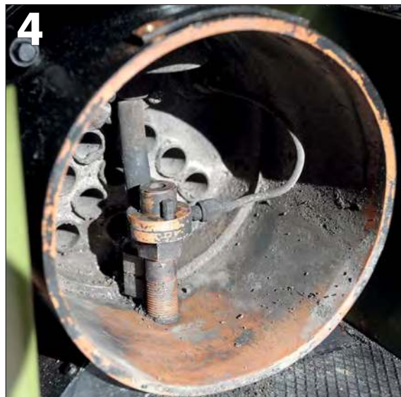
PHOTO 4: The completed blastpipe and blower arrangement.
