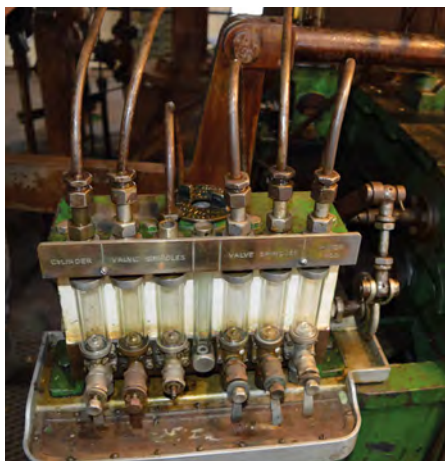
BELOW – The sight feed mechanical lubricator that feeds the cylinders, valve spindles and piston rods can be seen in this illustration. It was driven from the camshaft, although it is currently inactive on Engine No. 7.
