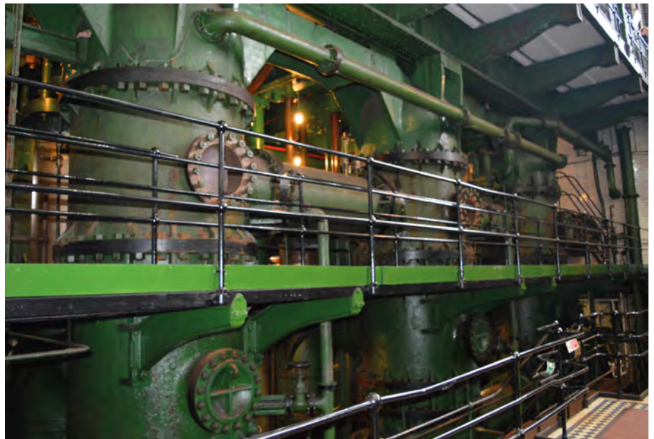
ABOVE The pumps worked by Engine No. 6.
