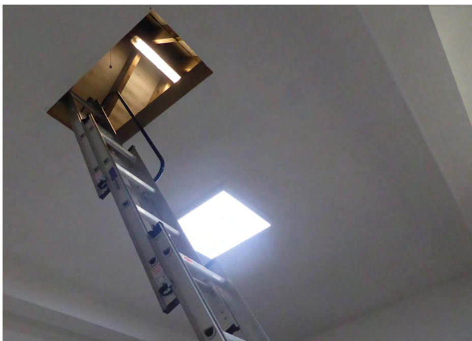
BELOW – PHOTOGRAPH 15 LED light panel in action.
