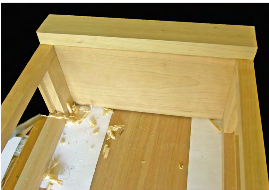
Photograph 60 – Protecting the rebates and fitting the top spacer piece.
