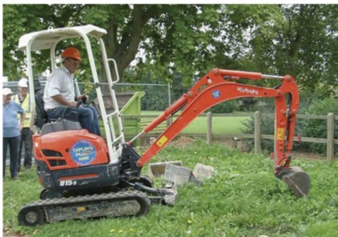
Cutting the first sod for the new City of Oxford S.M.E.E Clubroom.
