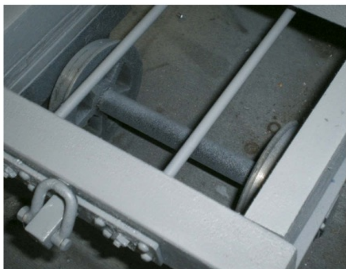
Details of the coupling shackle and iron work on the end beams.
