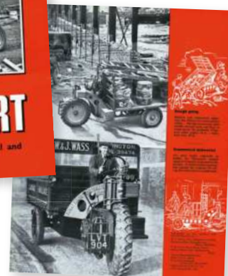
▼ The Motocart in use on a building site and an example used by a haulage company.
