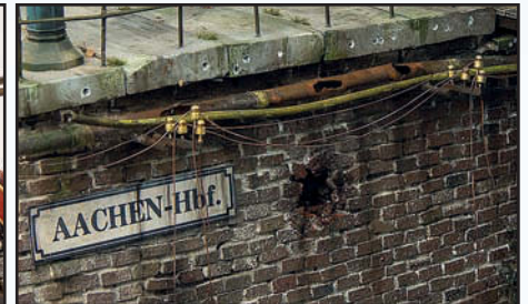
Here you can see the wires that were put on the insulators and the signs that were applied and weathered.
