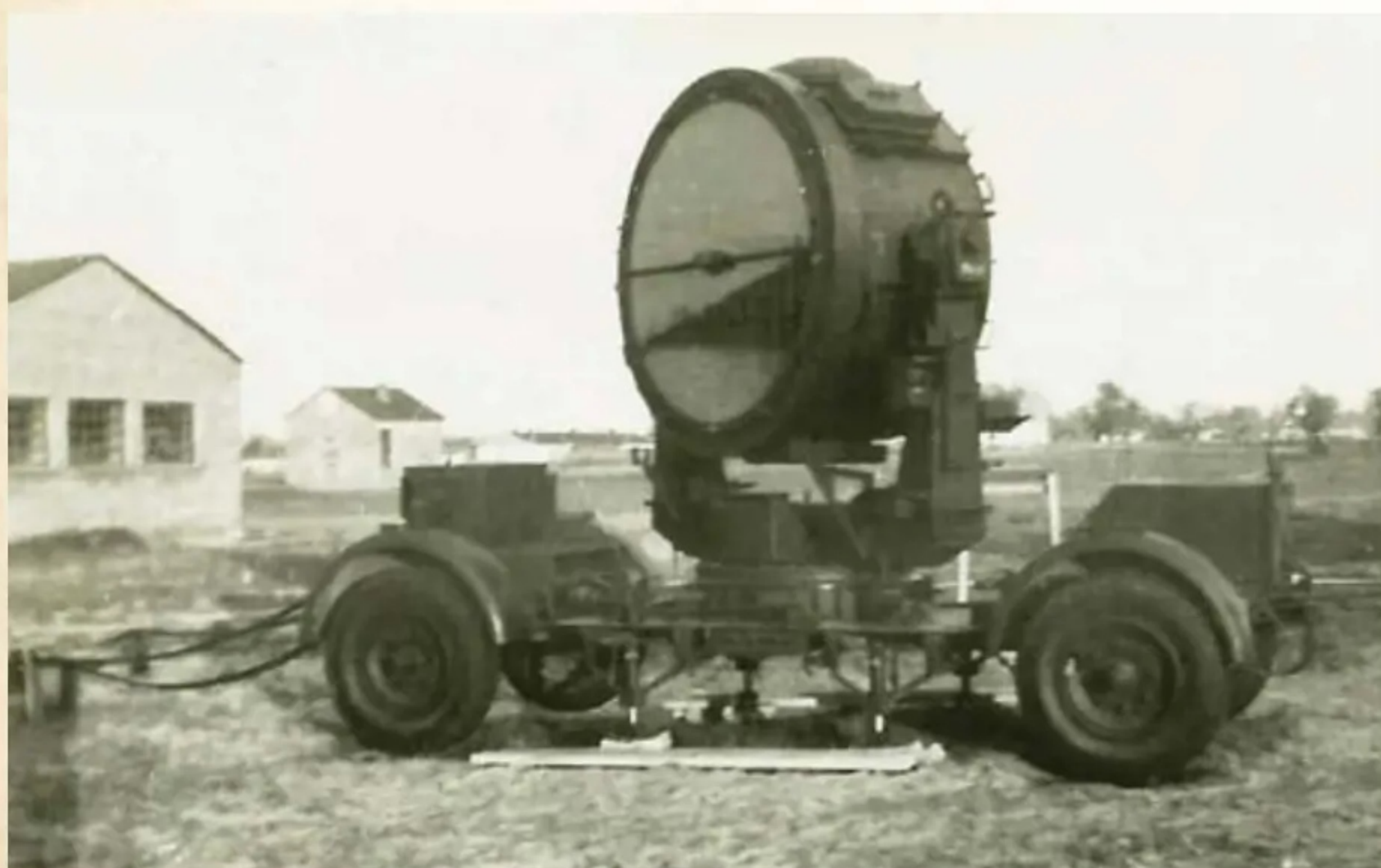
This is a profile shot of one of the few early style 150 cm Sw. 34 searchlights. This example is even rarer as it is one of the very few early 150 cm Sw. 34s to have stowage boxes mounted to the base trailer on both ends above the wheel axles and in-between the mudguards. The photo was taken within the perimeter of Frankfurt airfield in October 1940. It is worth noting that one of these very rare early 150 cm Sw. 34's with stowage boxes attached is on permanent display at Romania's military museum in Bucharest.
