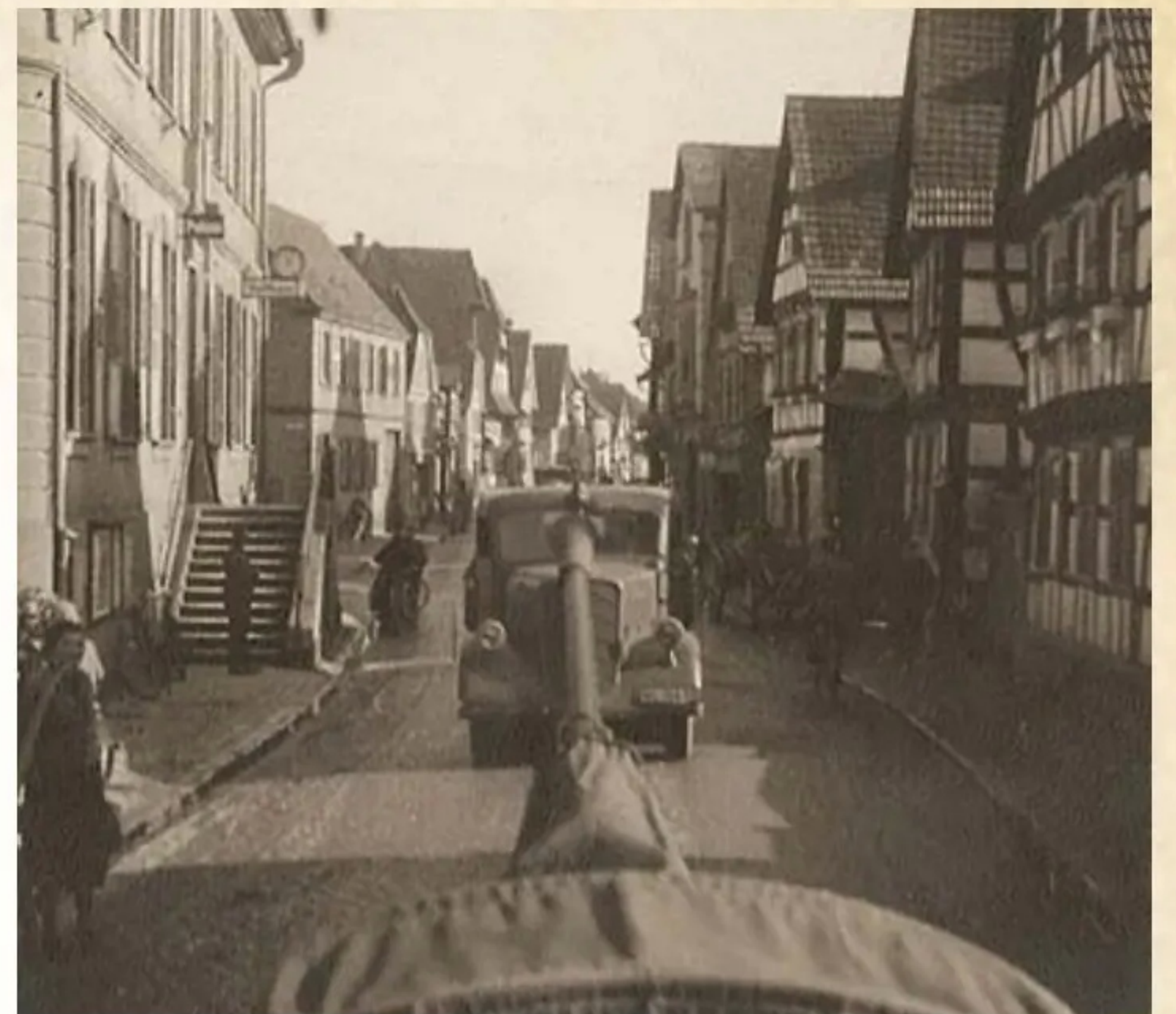
Elements of Luftwaffe Flak regiment 6 are pictured here travelling through Ghent, Belgium in the summer of 1940 sadly no date is given but I think looking at other photos taken in this series it was in late May or early June of 1940. The truck seen behind the barrel of a 37mm Flak gun is an Opel Blitz 2.5 ton type.
