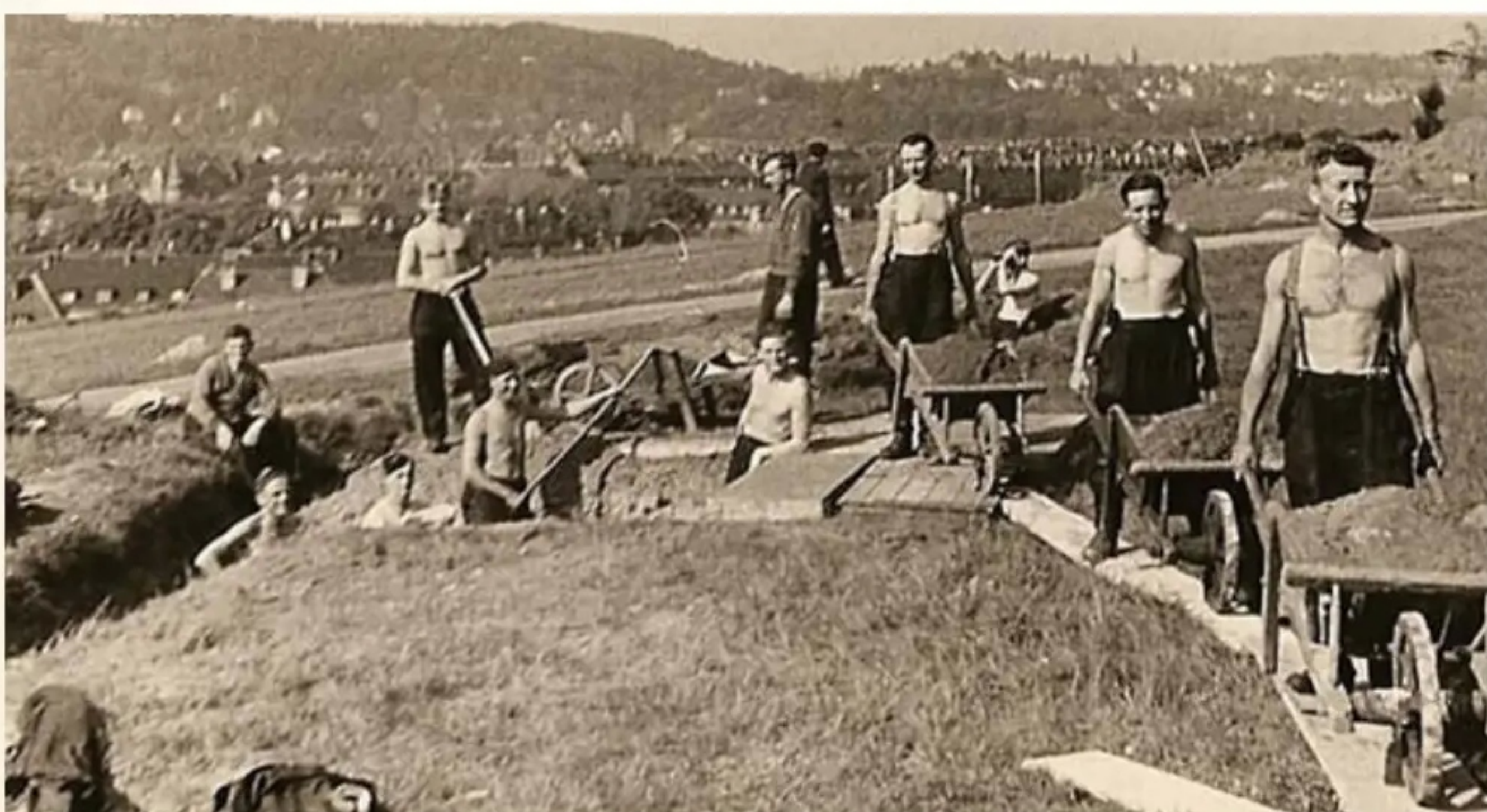
Here we have a photo of Flak troops from Luftwaffe Flak regiment 6 in the process of building a semi-permanent flak position in a hillside next to the channel coast in the summer of 1940. This position probably was later reinforced/expanded with concrete structures as part of the Atlantic Wall.
