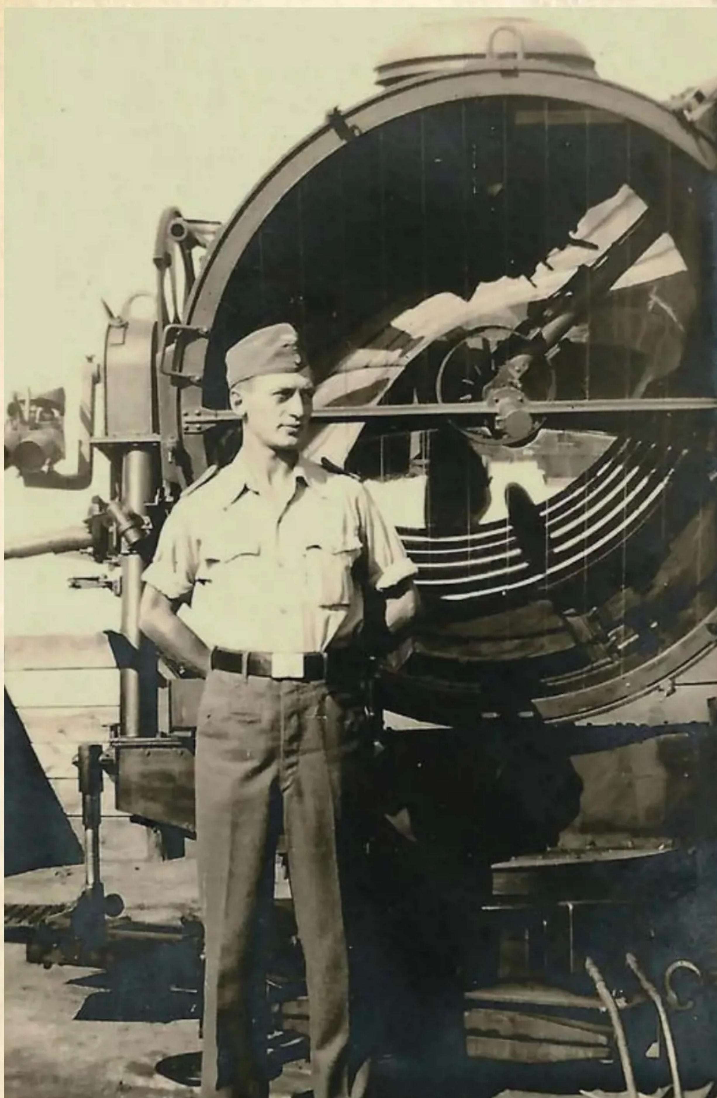
Above. A 150 cm Sw. 37 is used as a backdrop by a proud Leutnant (2nd Lieutenant) for his hero shot to send home in this photograph. A Doppelfernrohr 45° 10x80 Flakfernrohr is mounted on the side of the searchlight, which would have been used as a last resort to find/track a target if no targeting data or inaccurate targeting data was being supplied from other targeting/location equipment. The photo is dated July 1943, but no location is given.
