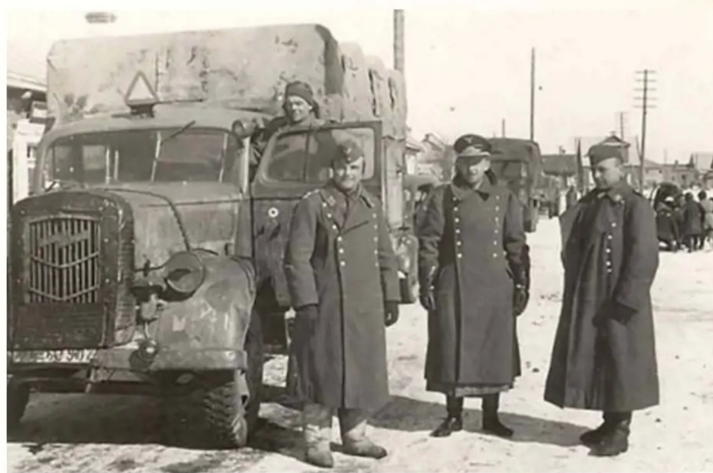
Photographed on in November 1943 in the Kraków area of Poland this photo shows us in the foreground an Opel Blitz 3 ton type 'S' belonging to the Luftwaffe. This ex-civilian truck still has its civilian number plate but has a Notek light fitted and an extra horn on the front bumper. A cold weather cover has been strapped over the radiator grill; it also has a small windscreen heater fitted. Lastly of note is that the truck is clearly not towing anything but does have its towing indicator triangle in the raised position.
