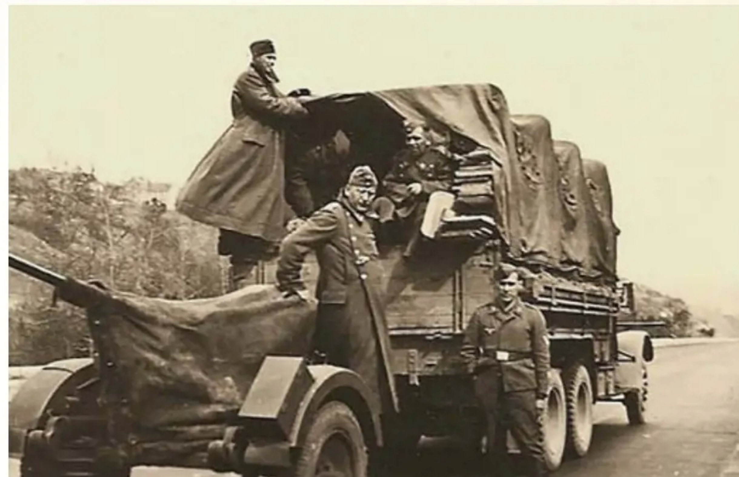
Another Henschel D33 that is seen here to be towing a 20mm Flak 30 mounted in its Sd.Anh 51 transportation trailer, photographed here on May 18th somewhere in Holland during the invasion of the west in 1940.
