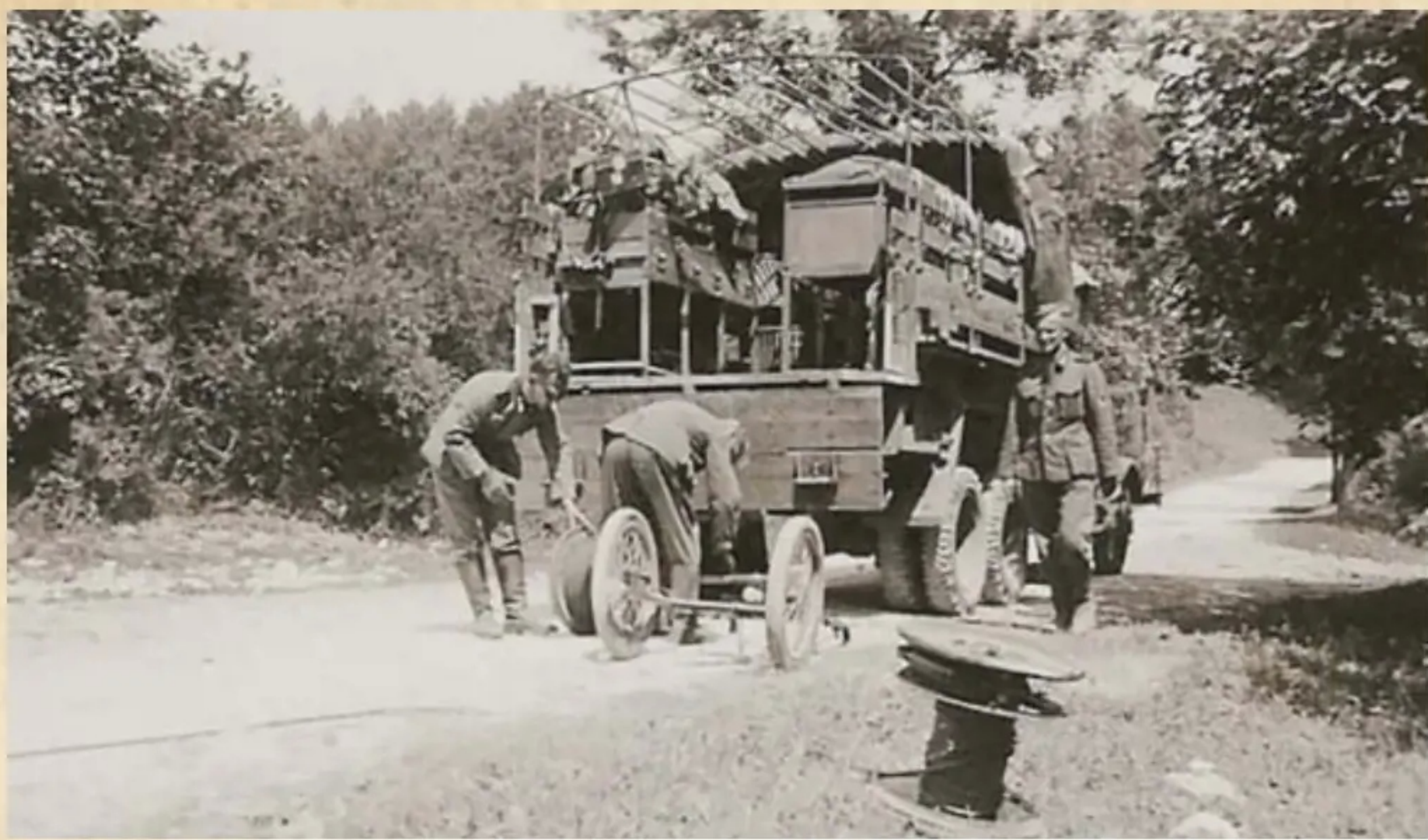
This Henschel D33 that belonged to a field telephone unit and is seen in the process of laying a long distance telephone cable along a French roadside in the latter stages of the invasion of the west in May and June of 1940. The photo was taken in the Alencon area south west of Paris during June.
