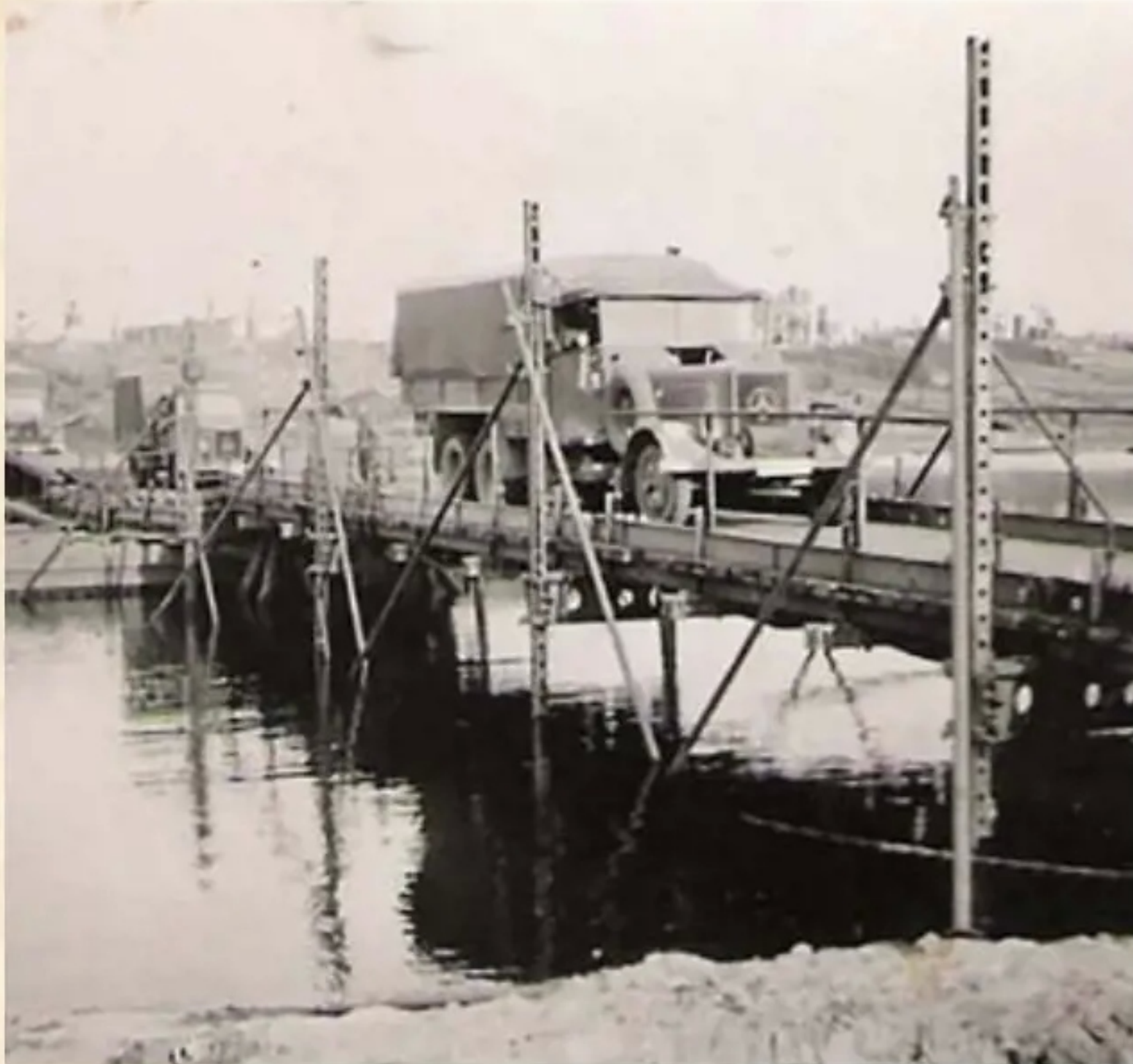
This Einheits-Diesel was photographed crossing a German pioneer's prefabricated field engineering bridge that was erected to cross the River Meuse south of Sedan during the 1940 invasion of France. The photo was taken in late May of that same year.
