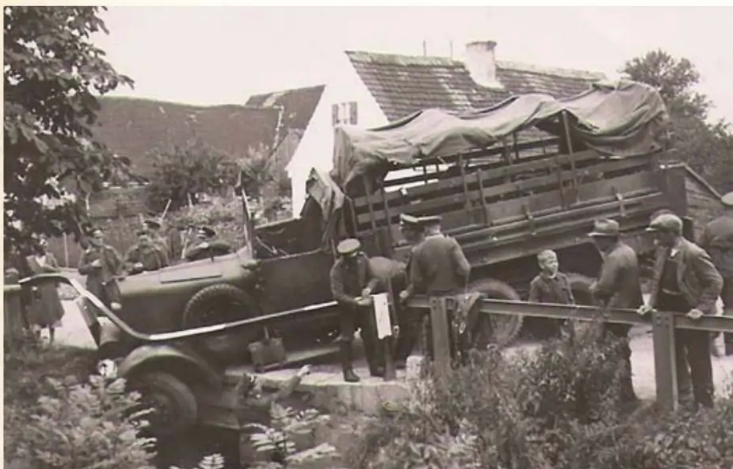
A Mercedes-Benz LG 3000 that has not been able to manage the turn radius required to negotiate this road junction, and has pushed through the barrier and over the edge of a drainage culvert. This accident happened on the 24th of August 1941 close to Metz in Eastern France.
