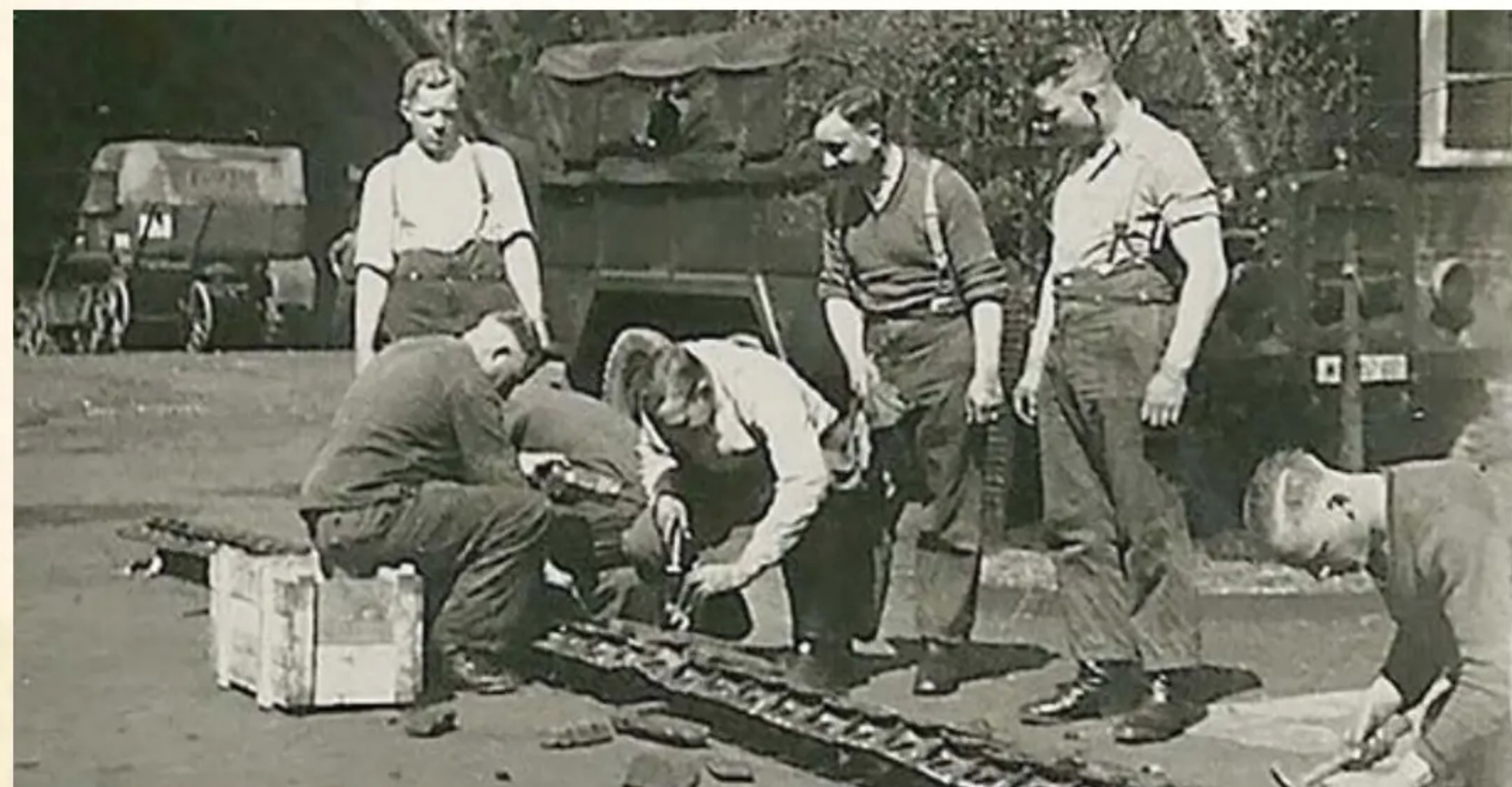
In the same commandeered French farm yard as mentioned earlier on this page we see maintenance crew giving the tracks of an Sd.Kfz 7 a thorough going over no doubt cleaning the tracks replacing all the damaged Greece nozzles and lubricating all the as required this took quite a while and was the most time consuming regular maintenance task on the normal crew task list and was rarely carried out with as much diligence as it should have been hence scenes like this.
