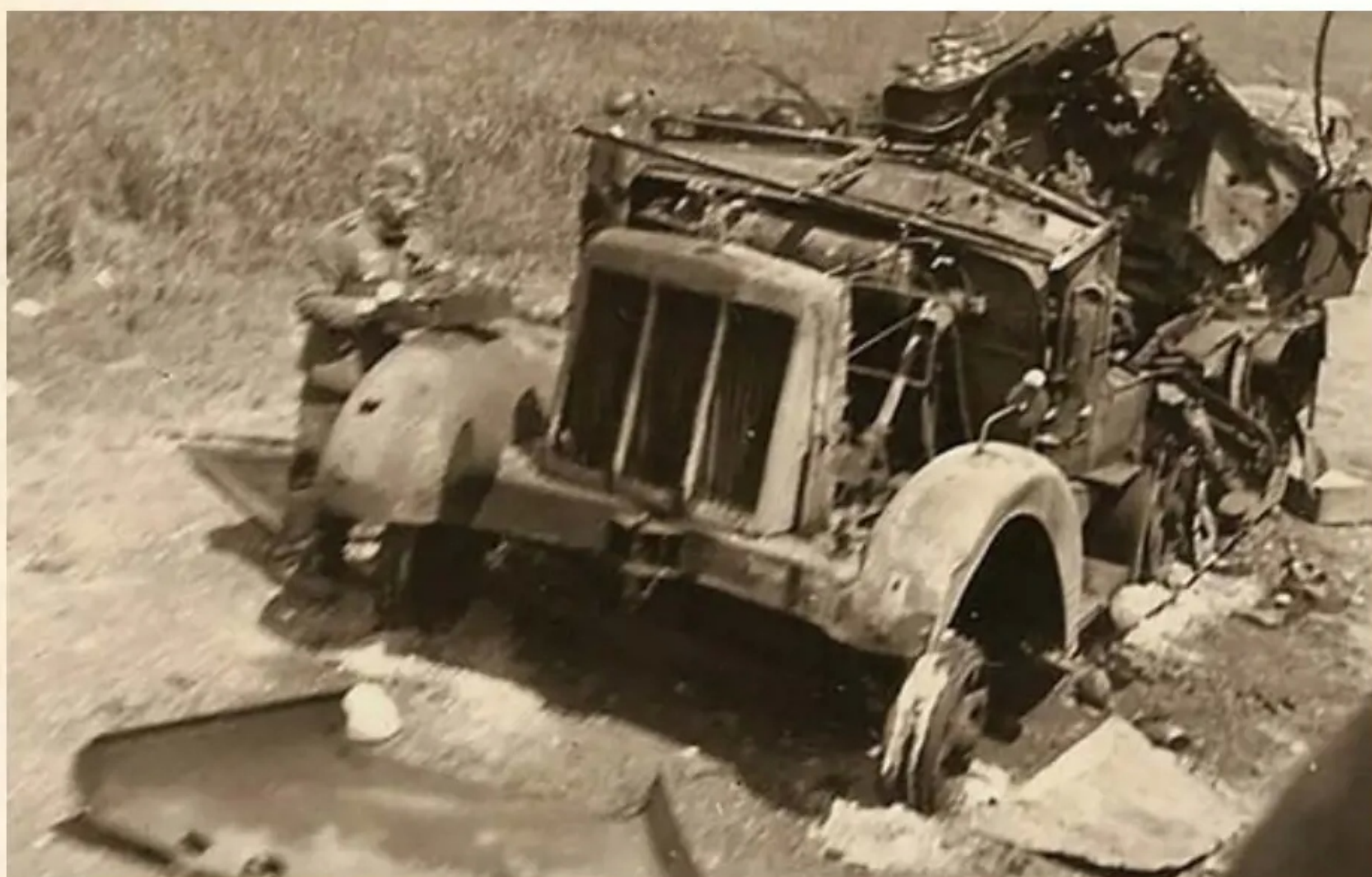
Photographed on the June 1st 1940 this Sd.Kfz has fallen fowl of an anti-tank mine unfortunately for the Sd Kfz 7 whilst the front wheels passed over the mine without issue the halftrack section did not and being unarmoured as opposed to the mines intended target of a tank the damage the mine caused was catastrophic.
