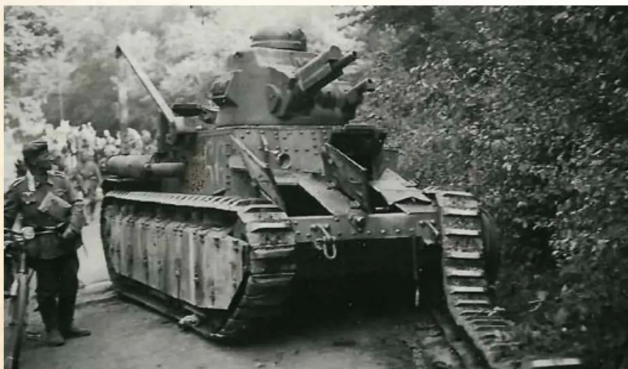
The location is only very vaguely given here as a few kilometres west of Reims. Again I do have a date, this photo was taken on the 14th of June 1940 and the caption tells of how this Renault D1 was put out of action by as many as 14 shots from 37mm Anti-tank guns into its left flank.
