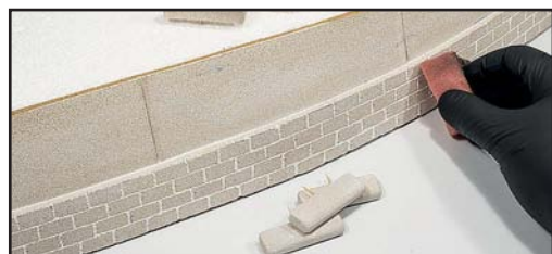
It also gets a coat of wall filler squeezed between the rocks, and smoothed out using a wet sponge.
