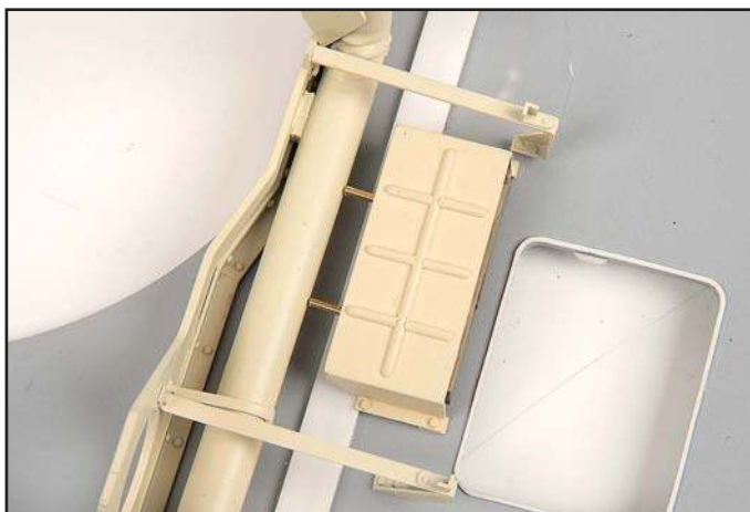
The pre-painted box and tray were glued together and a pair of 1mm brass pins were drilled through the back of the tray into the box and glued into position. Their location on the roof was established.
