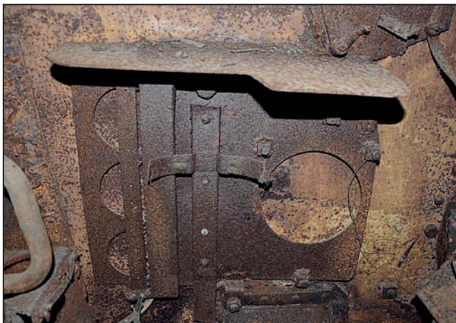
On the Hull wall next to the Driver's seat is this bracket with its protective lip. It took some detective work to work out the exact purpose of the bracket. I knew that the left hand side contained the fuse panel as I had seen this
