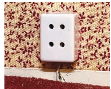
Outlet glued in place. Cover wire with baseboard.
