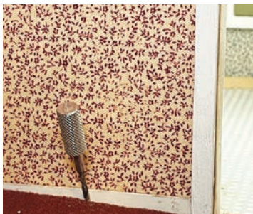
Drill a hold at the bottom of the baseboard.
