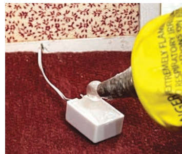
Apply glue to the back of outlet and position to wall.
