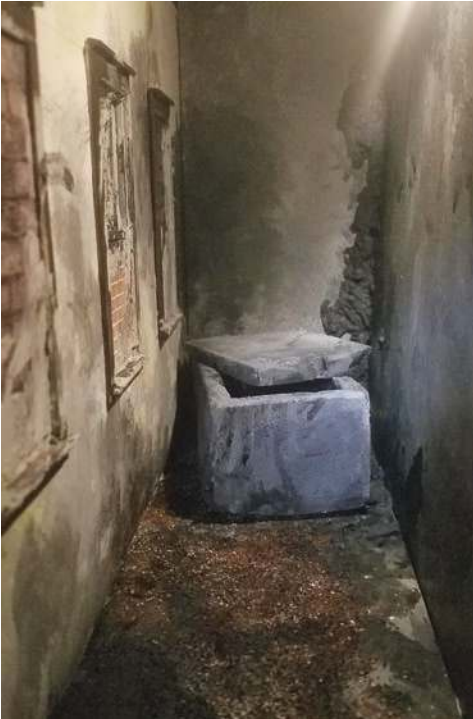
Above: The windows in the dark dusty crypt are filled in with bricks.
