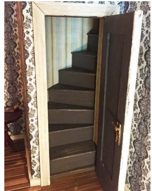
Above: The attic stairs were built in as a false wall insert.
