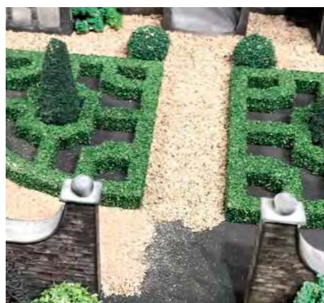
▲ Gravel paths under construction
