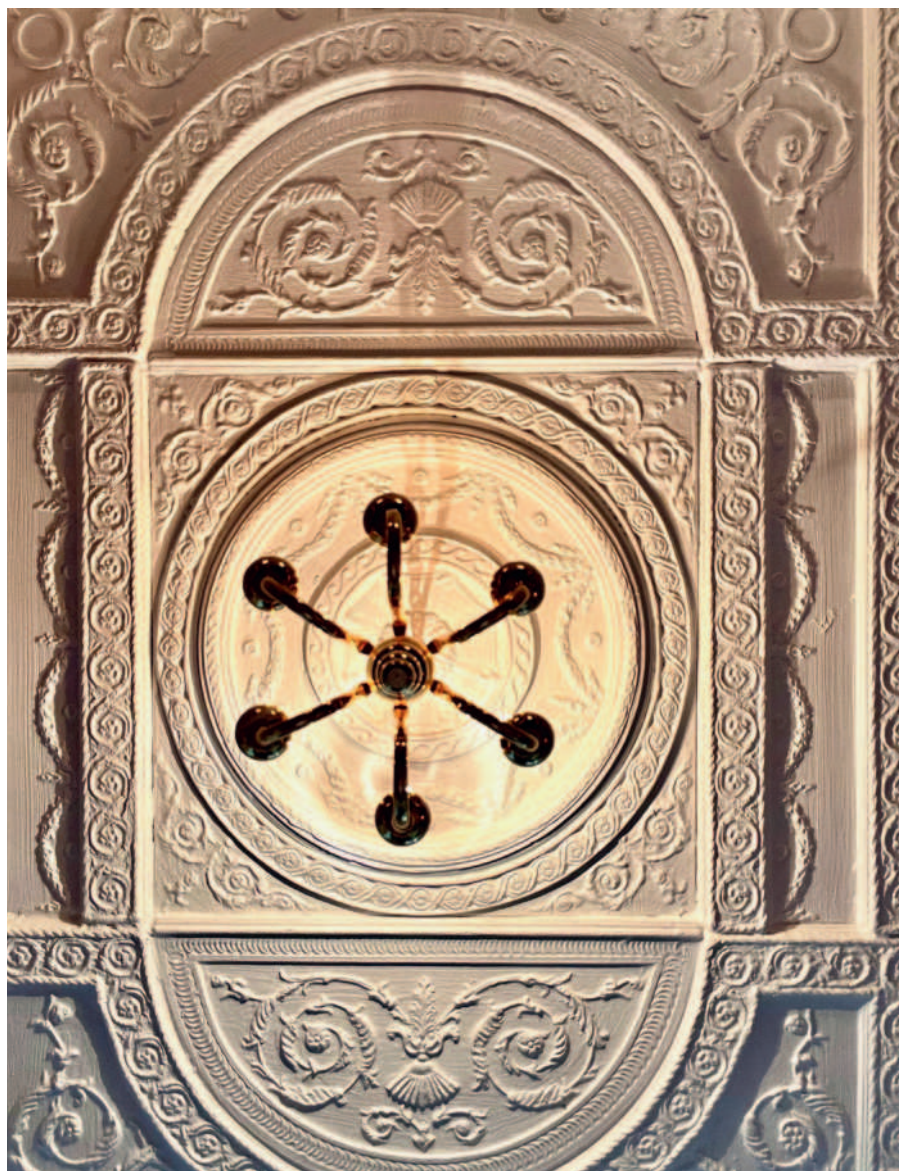
▲ Spectacular plaster ceiling
