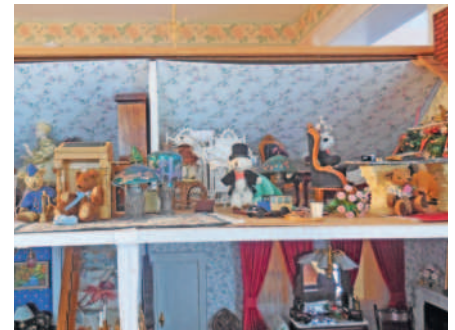
▼ BEFORE - Sagging ceilings
