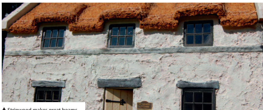
▲ Stripwood makes great beams
