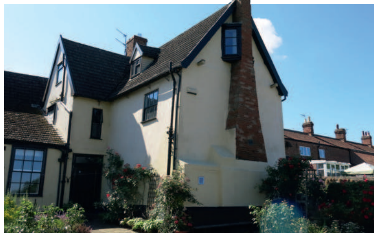
▼ 16th Century timber framed Hamblyn house rear view
