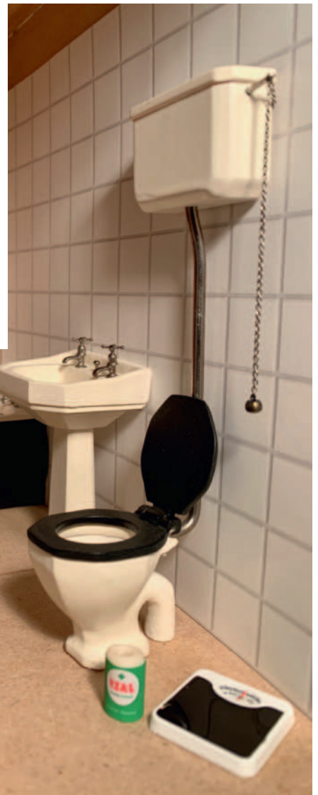
▼ Moi's bathroom awaiting tiles and flooring
