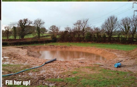
When infilling, pay attention to the gradient of the pond's sides
