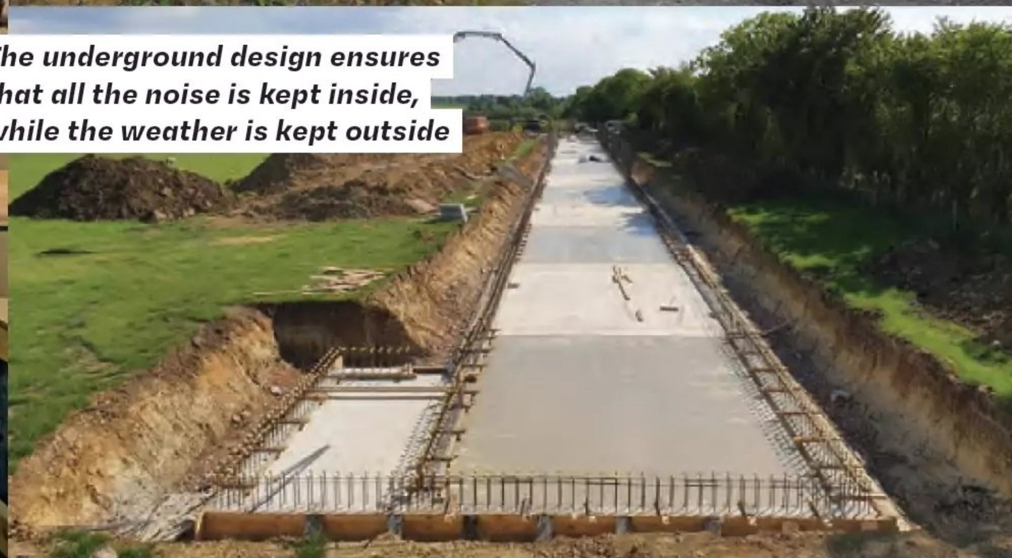
Although the 100m range is operational, there is still a lot of work to be done before the whole facility is ready
