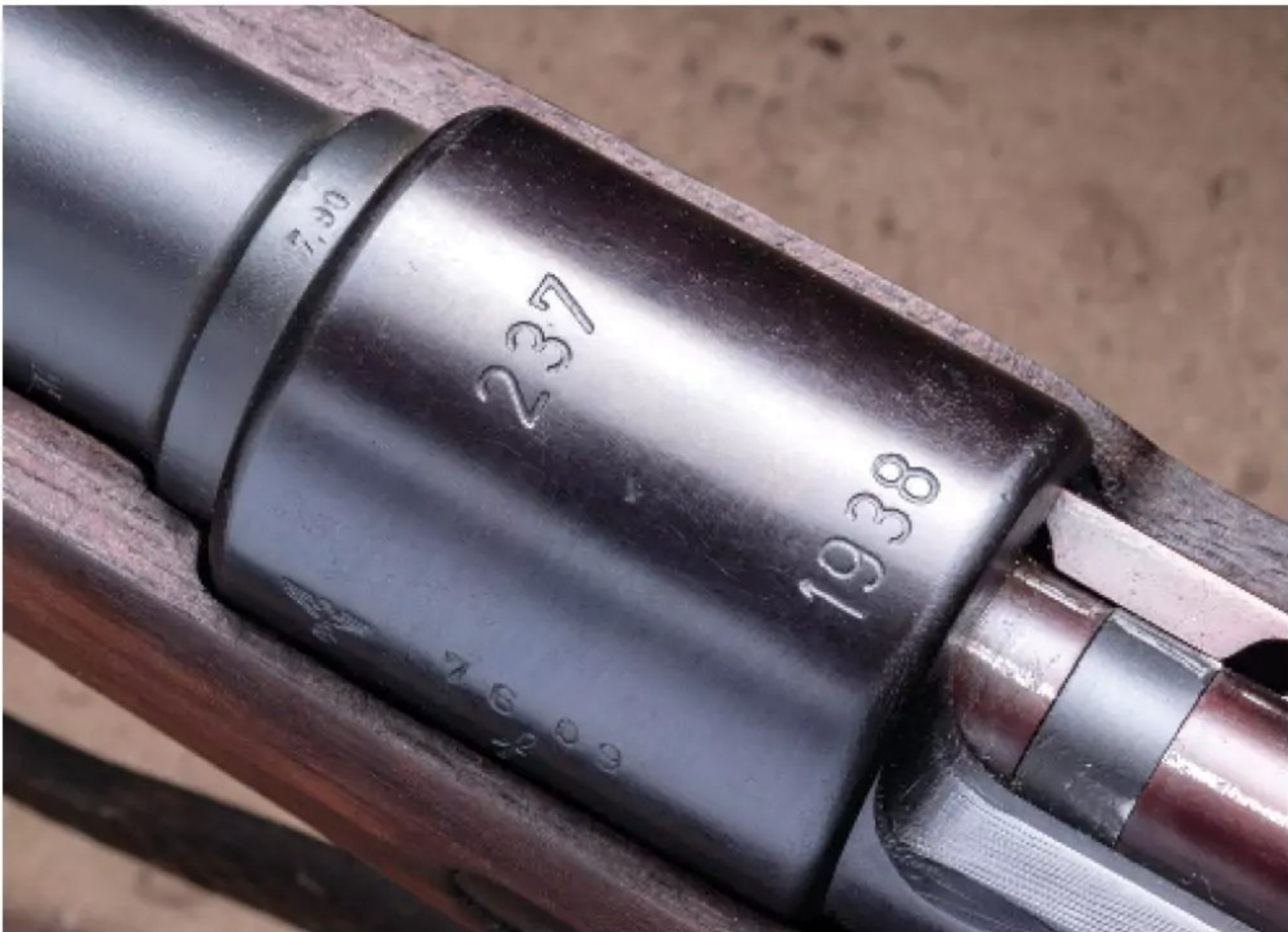
The manufacturer code and production date can be accompanied by the caliber marking on the receiver bridge.
