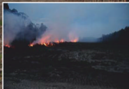
Stump removal in progress at the site.
