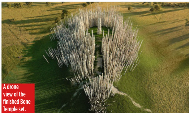
Over 900 uprights were sunk into rocky ground.
