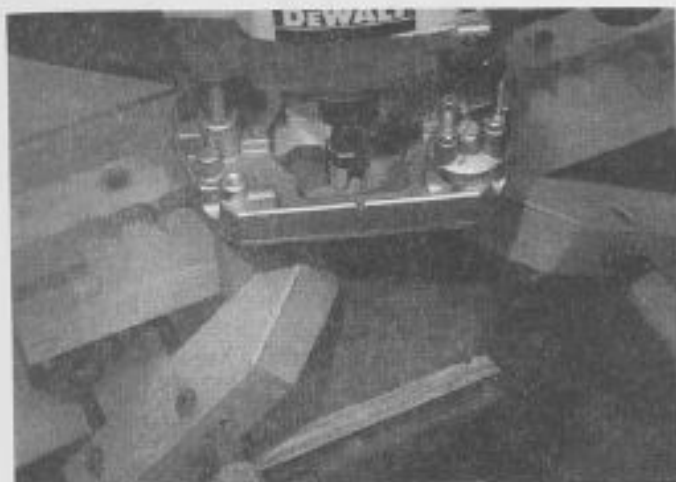
18-47. ▶ The routing operation.
