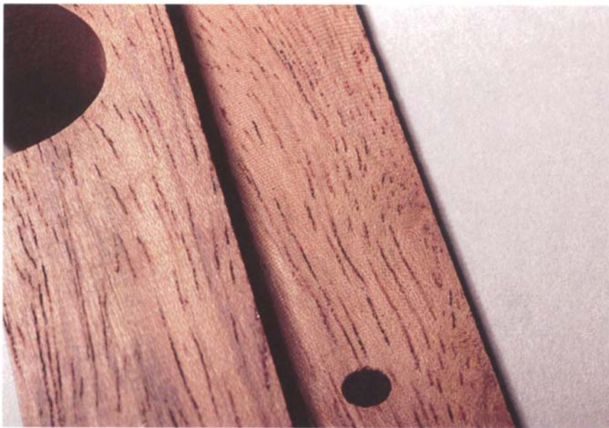
The floor of this rabbet shows the slight swirls of the cutter tip. The wall is typically much cleaner than the bottom cut.
