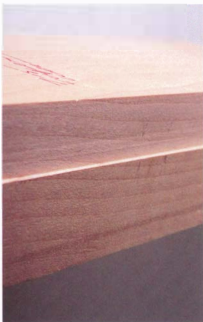
Close inspection reveals the cutter wear line on the work. The slight step will frustrate or prevent a close-fitting joint.
