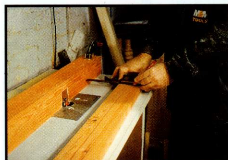
▲ Mark the moulding lengths across the spindles
