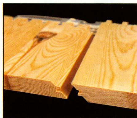
Using a lock mitre to make up a wider board
