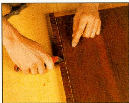
Lay the next piece, then cut through both to make the join
