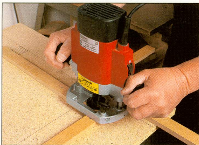
▲ The hole being routed using the sticks as a guide rather than the template
