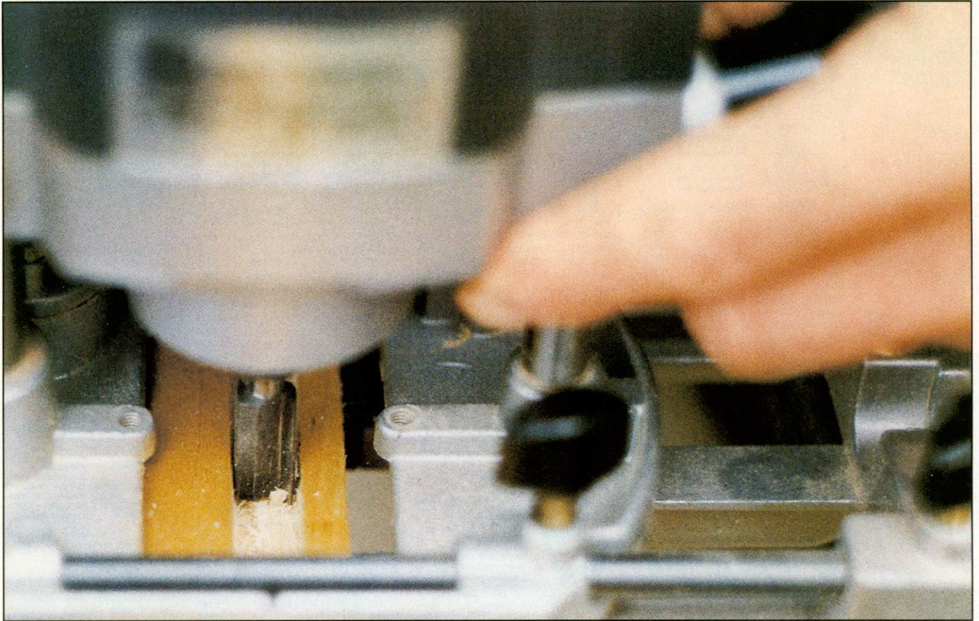
▲ Routing the groove for the rebated boarding
