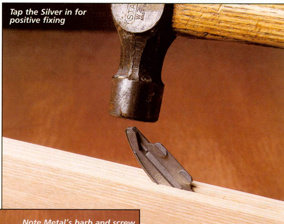
▲ The S-Klick clips straight in to mount small sections
