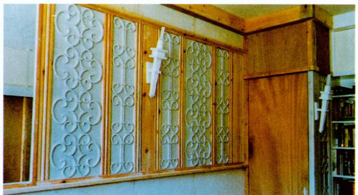
Parts fixed to the panel by veneer pins
