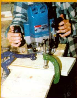
Cut grooves before shaping ends
