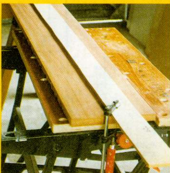
Using rod to mark uprights
