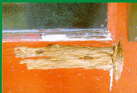
Beading and glass removed
