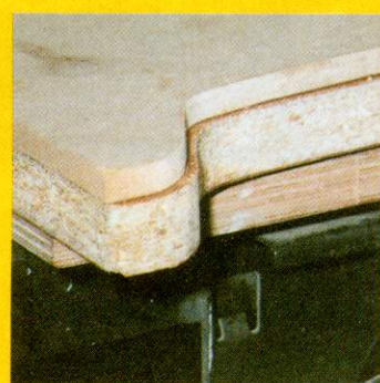
Shaping bottom of centre upright C or D
