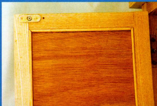
Door of chest showing magnetic catch part and beading retaining panel
