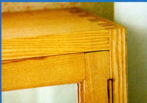
Chest, showing bottom lap dovetails
