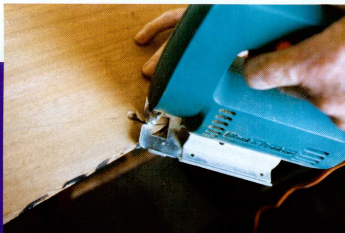
6. Jigsaw being used to cut shape of side, with hole drilled to facilitate change of direction of jigsaw.
