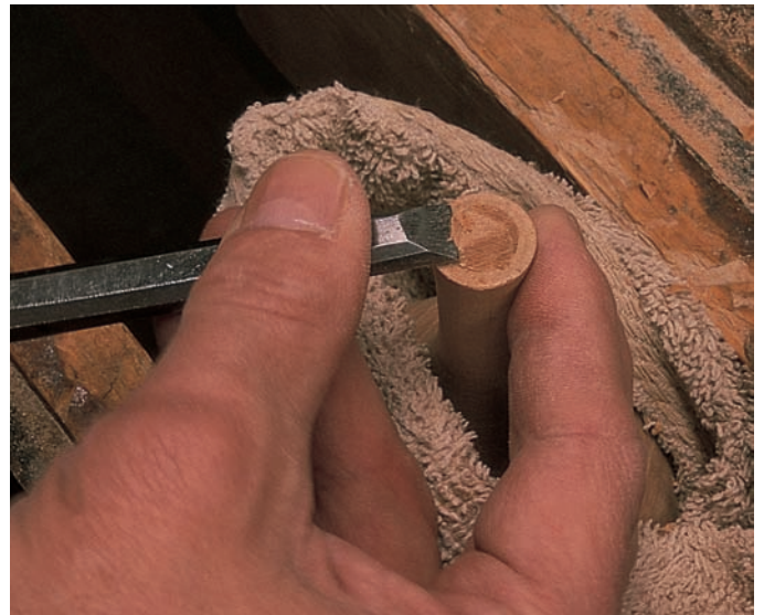
step 12 With a sharp chisel, pare away the excess just below the saw cut.
